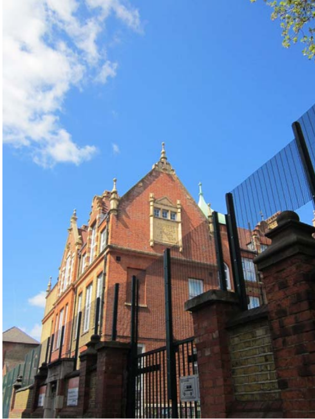
Figure 3: Princess May Primary School
