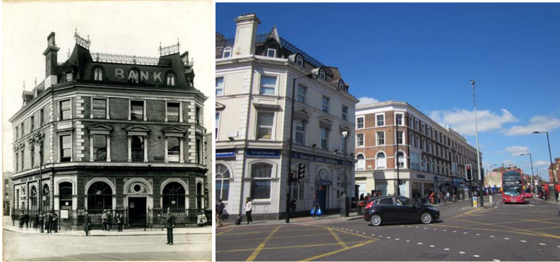
Figures 32 & 33: No. 1 Kingsland High Street in 1930 and No. 1 and Nos. 3-23 Kingsland High Street
