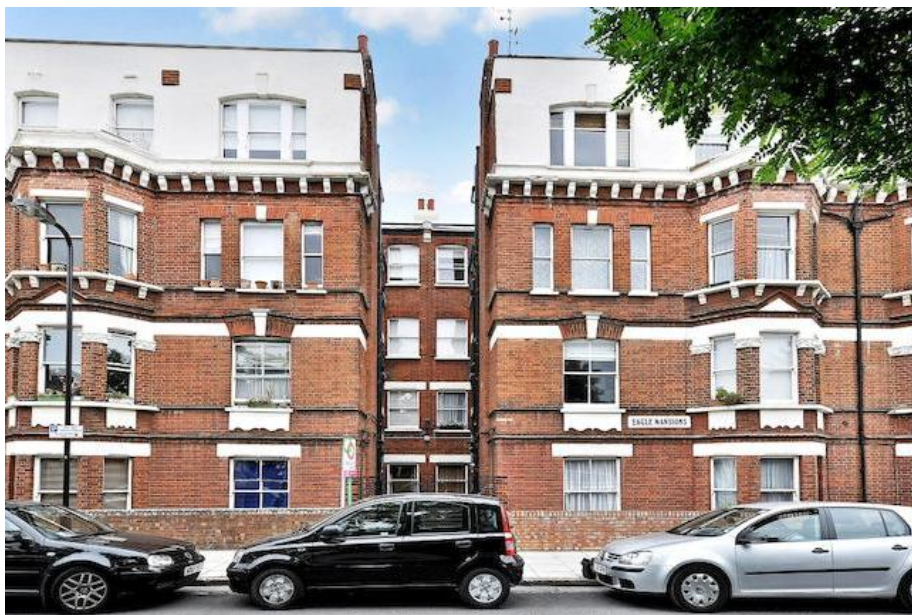
Figure 50: Eagle Mansions, Salcombe Road
