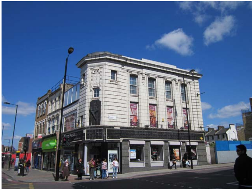
Figure 1: No. 2 Kingsland High Street looking north
