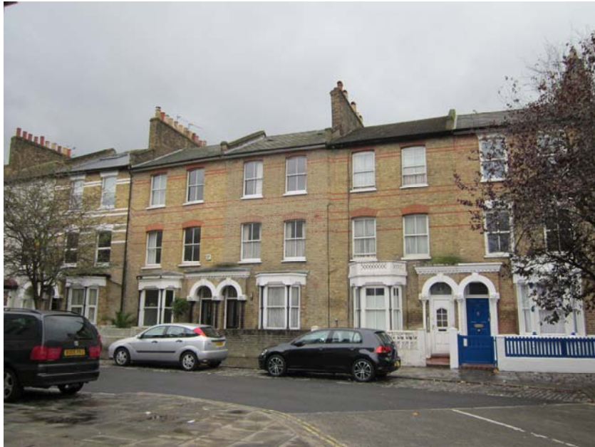
Figure 48: Nos. 23-31 John Campbell Road
