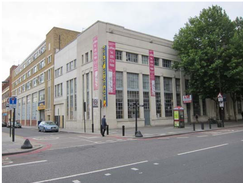
Figure 30: The former Simpson's Factory of 1929
